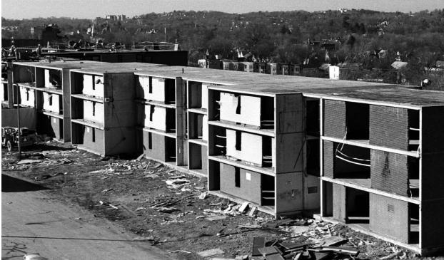
The original Academy Homes II included buildings up to nine stories high with no elevators, and weak, failure-prone slab support structures. Tenants found housing elsewhere while the original project was demolished, and many have been able to return to the replacement units.
