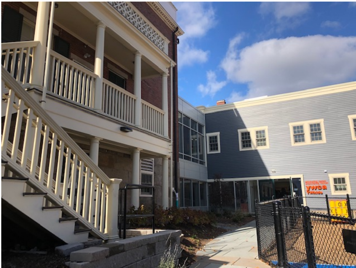
The rear of the building features a dedicated entrance to the afterschool program (right-hand side), outdoor place space, and a seamless connection to the original building (left-hand side).
