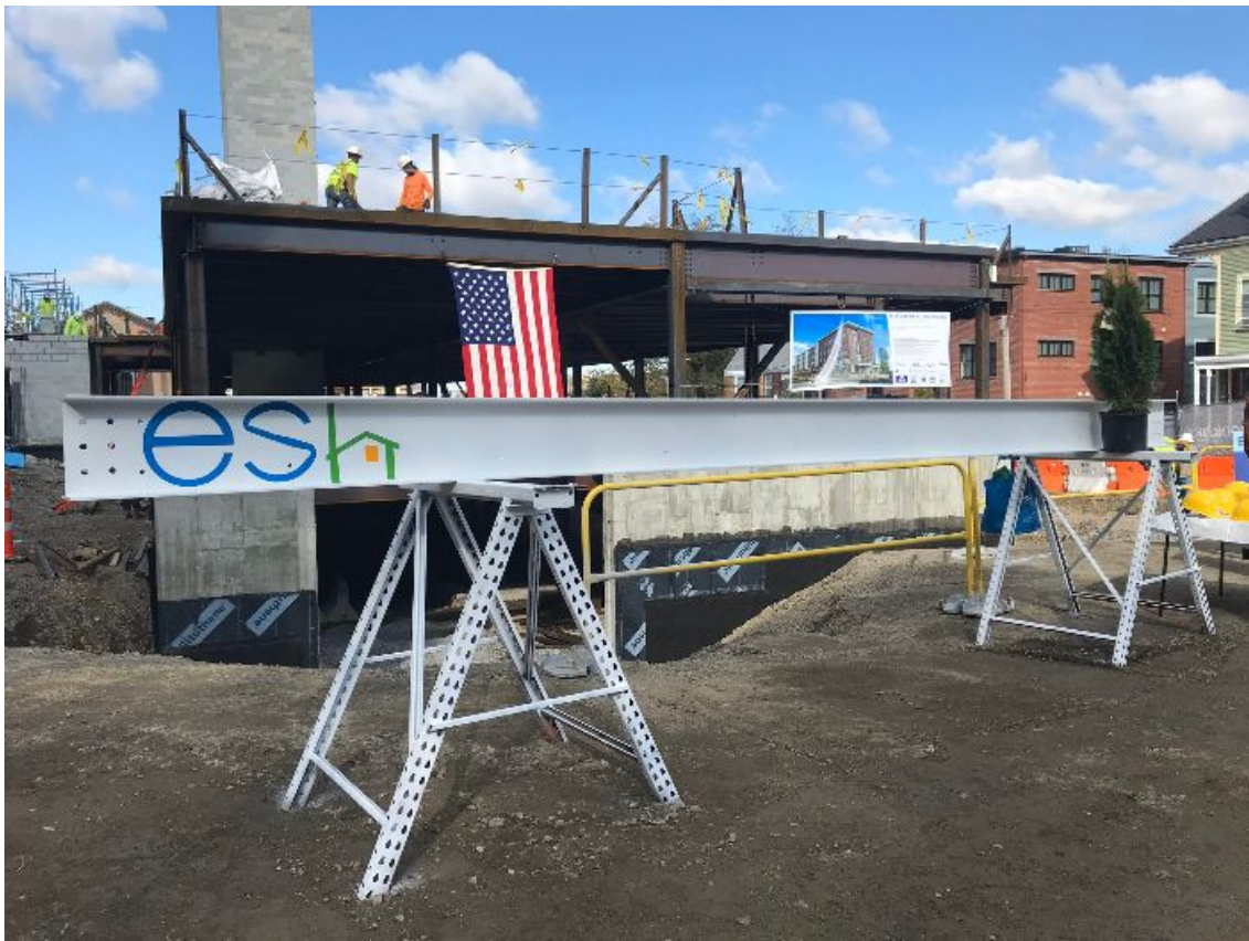
Final steel beam marking the "Topping Off" of the building's frame.
