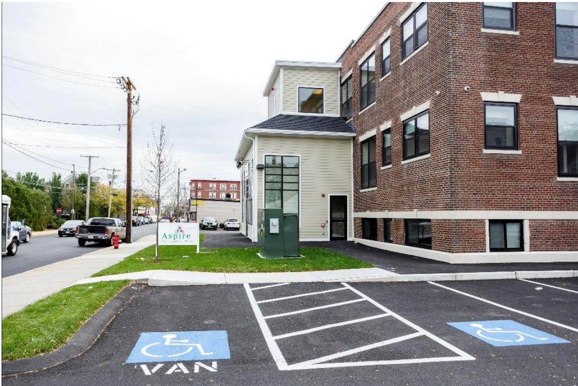
Accessible parking spaces and entrance at Aspire Developmental Services in Lynn, MA.
